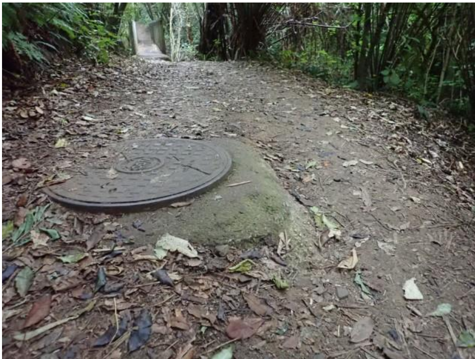
Photo 15: Sewer pipe cover
