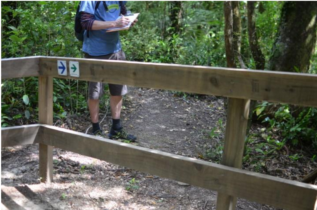
Photo 1: Barrier across track (near 800-year-old rimu)
