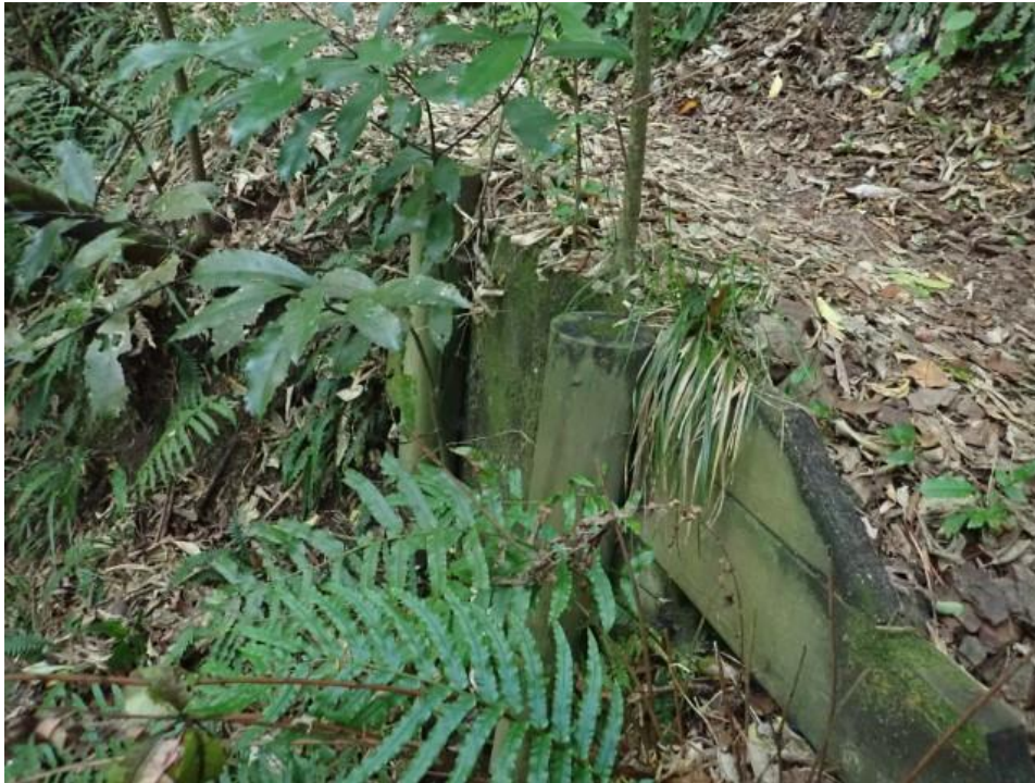
Photo 15: Retaining wall – 2 metres long and 1.5 metres high
