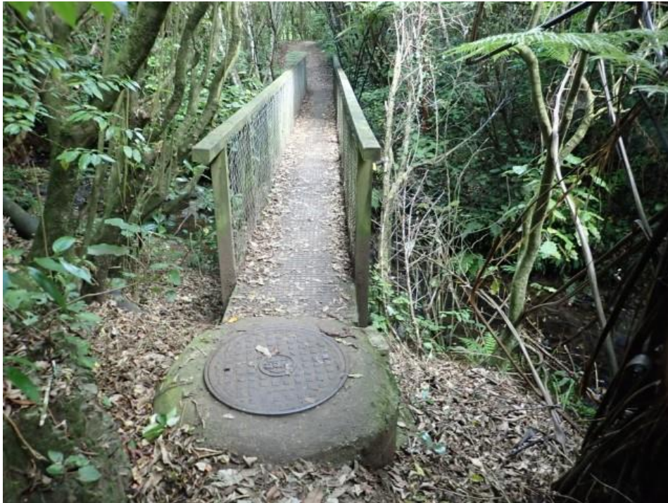
Photo 16: 15-metre-long narrow bridge – 0.78 m with wire sides
