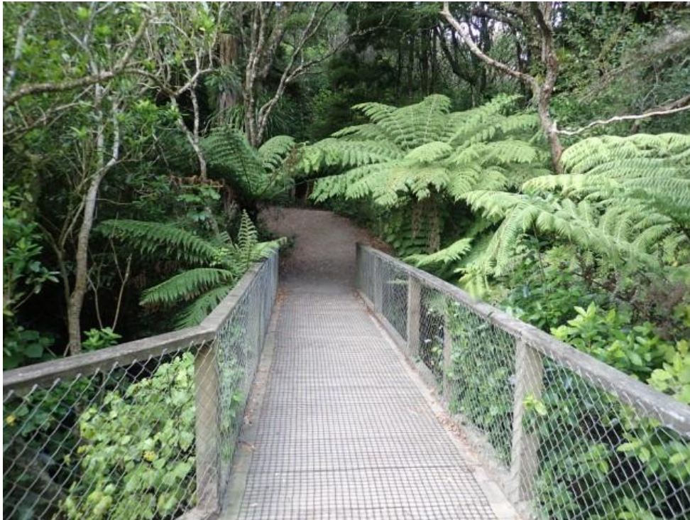
Photo 18: Bridge at northern end of the Troup Picnic Area
