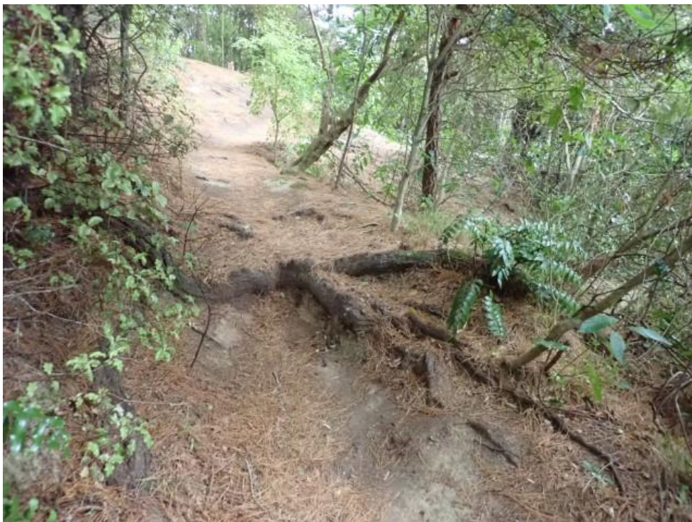
Photo 6: Large root with drop below Comment: It is difficult to tell how big this step down is from above. Recommendation: Construct 4 box steps down from the root.
