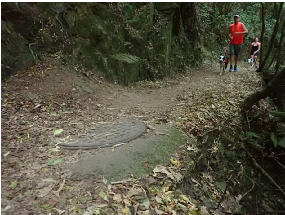
Photo 11: Pinch point at sewer pipe cover
