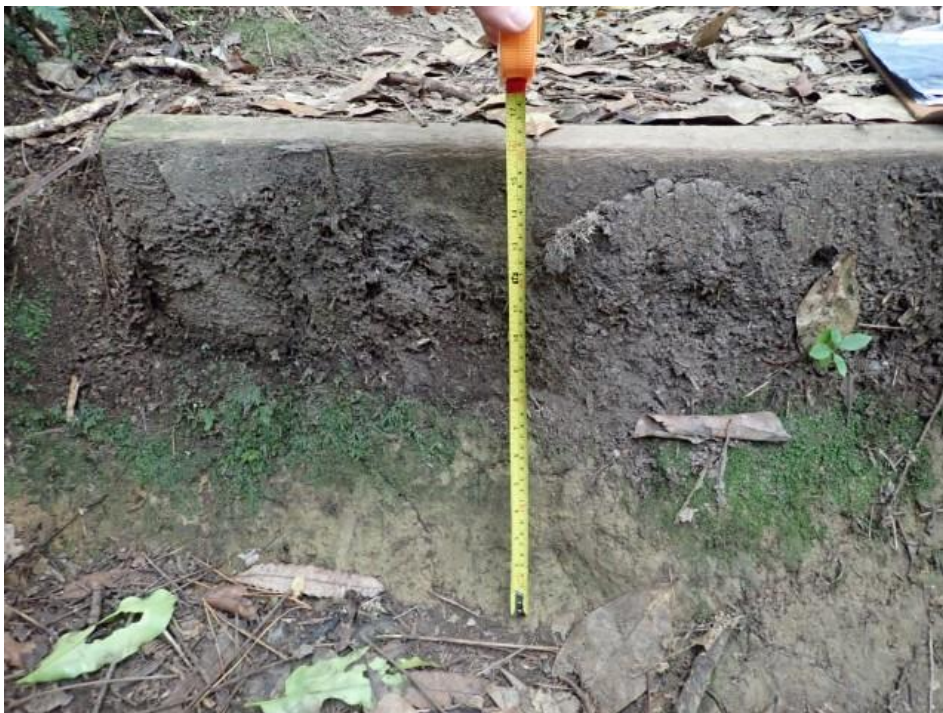
Photo 10: 420mm riser (200mm wood and then soil compaction over 15 years)
