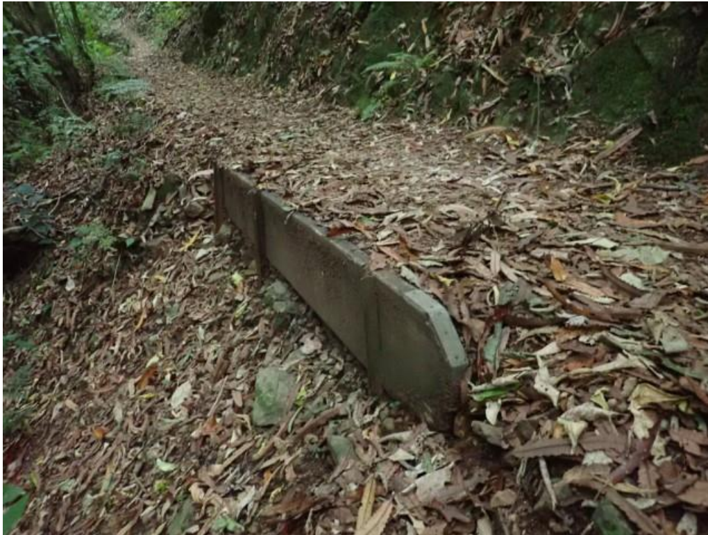
Photo 17: Minor retaining board – 3 metres long
