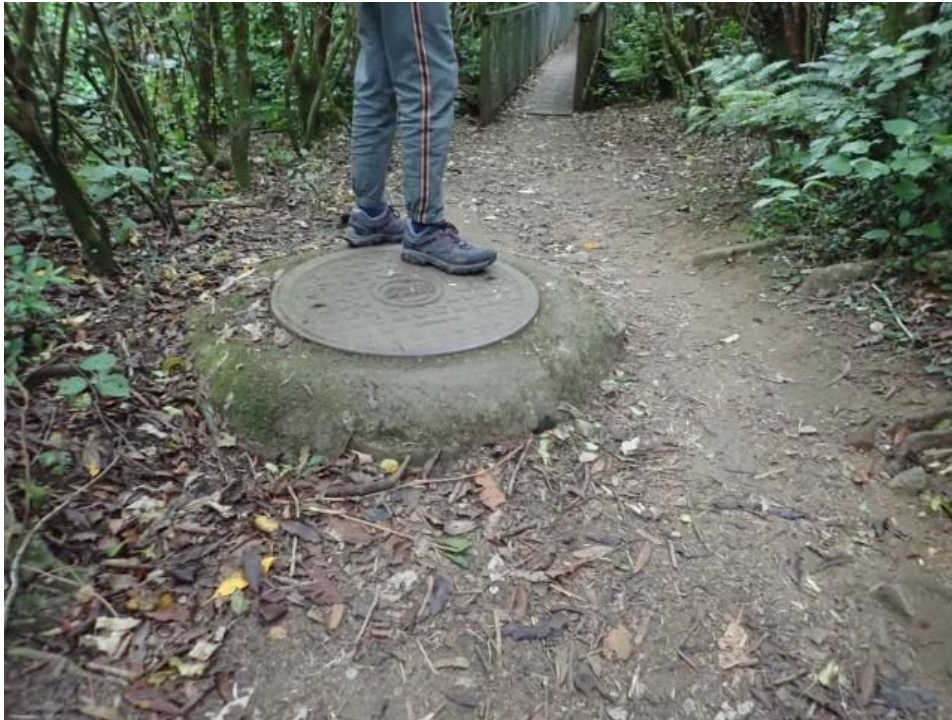
Photo 18: Sewer pipe cover
