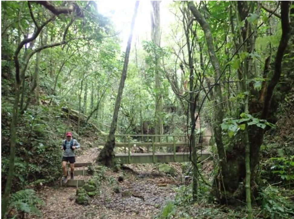
Photo 37: 3 steps and bridge (6 metres by 0.9 metres, with 20 years remaining life)
