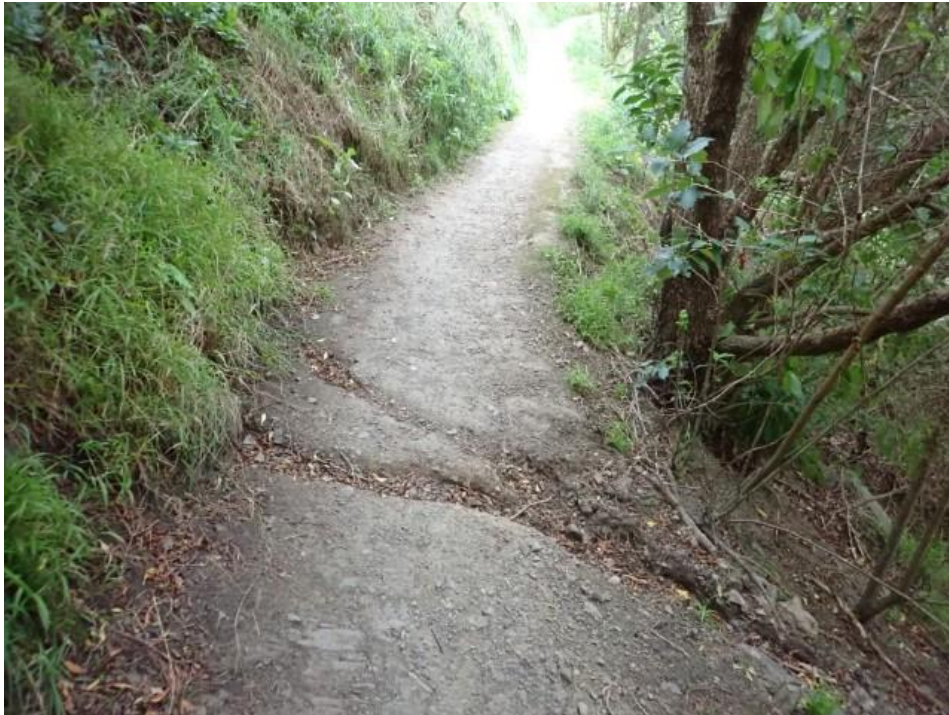
Photo 30: Water runnel across the track
