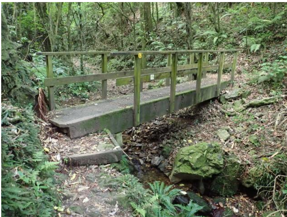
Photo 38: Bridge and step
