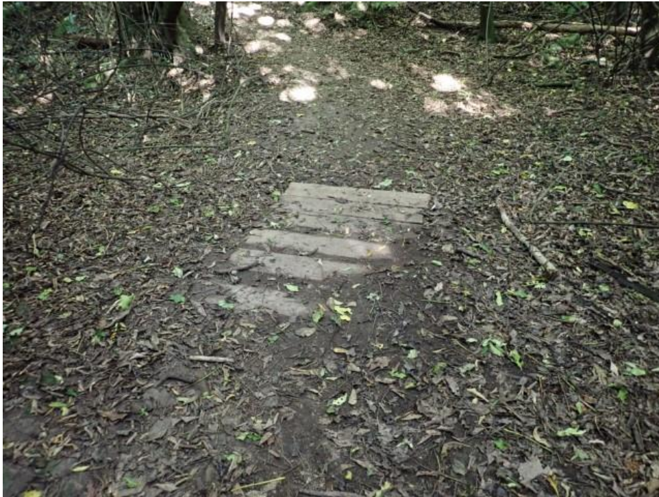
Photo 21: Submerged 1.5m long boardwalk
