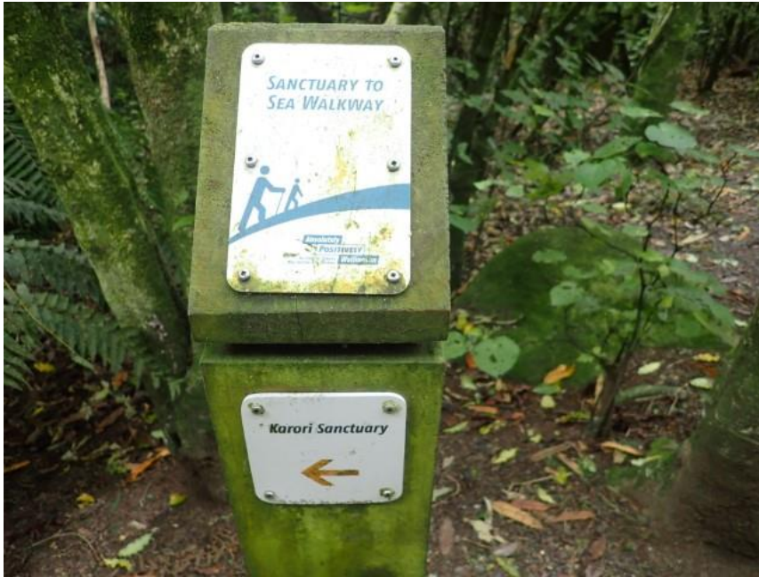
Photo 45: Dirty bollard signs
