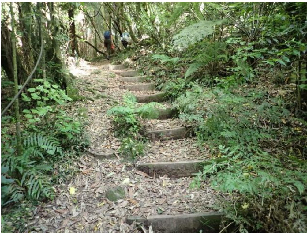
Photo 47: Start of 24 steps steeply uphill out of gully Comment: Could be avoided as terrain is not difficult. Recommendation: Investigate a reroute.
