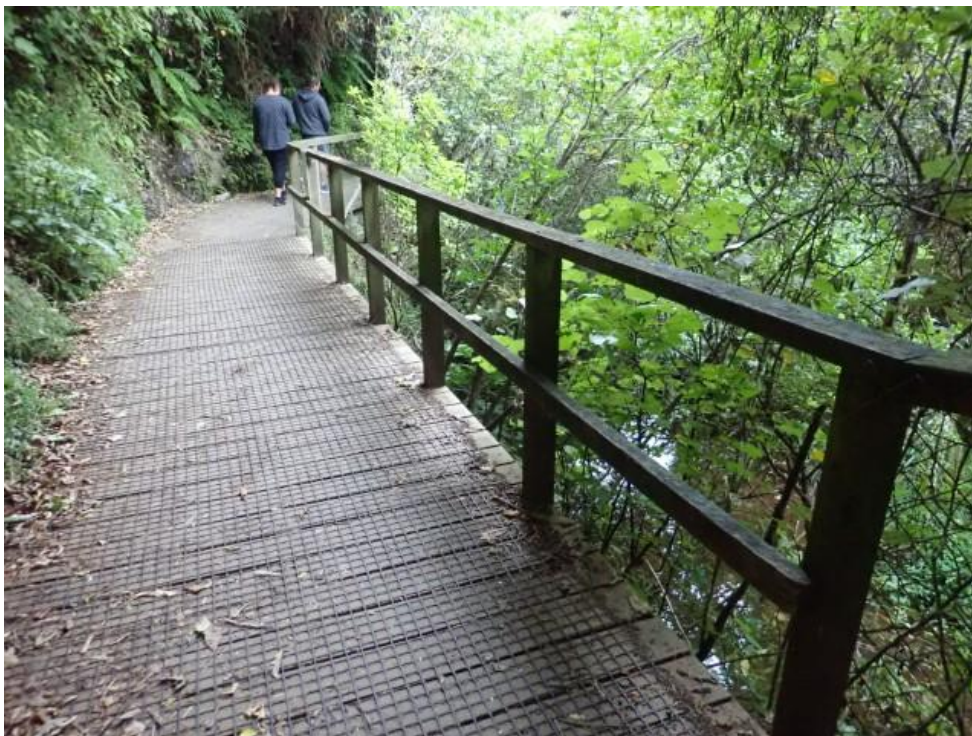
Photo 5: 30 metre boardwalk beside stream.
