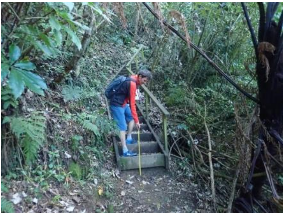
Photo 4: Large step at bottom of the last flight with a handrail
