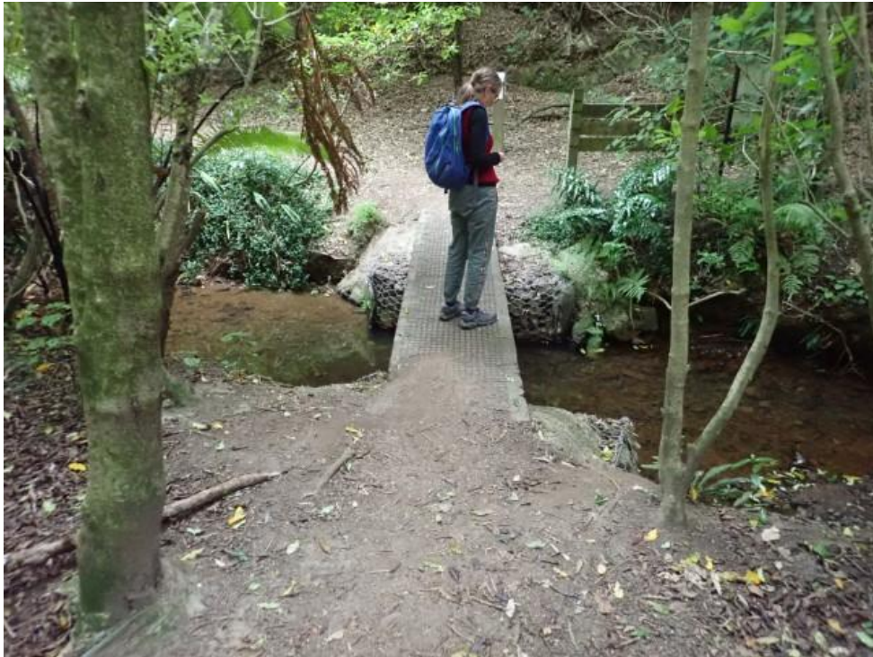
Photo 11: The bridge over Kaiwharawhara Stream
