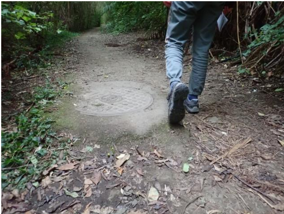
Photo 13: Sewer pipe cover
