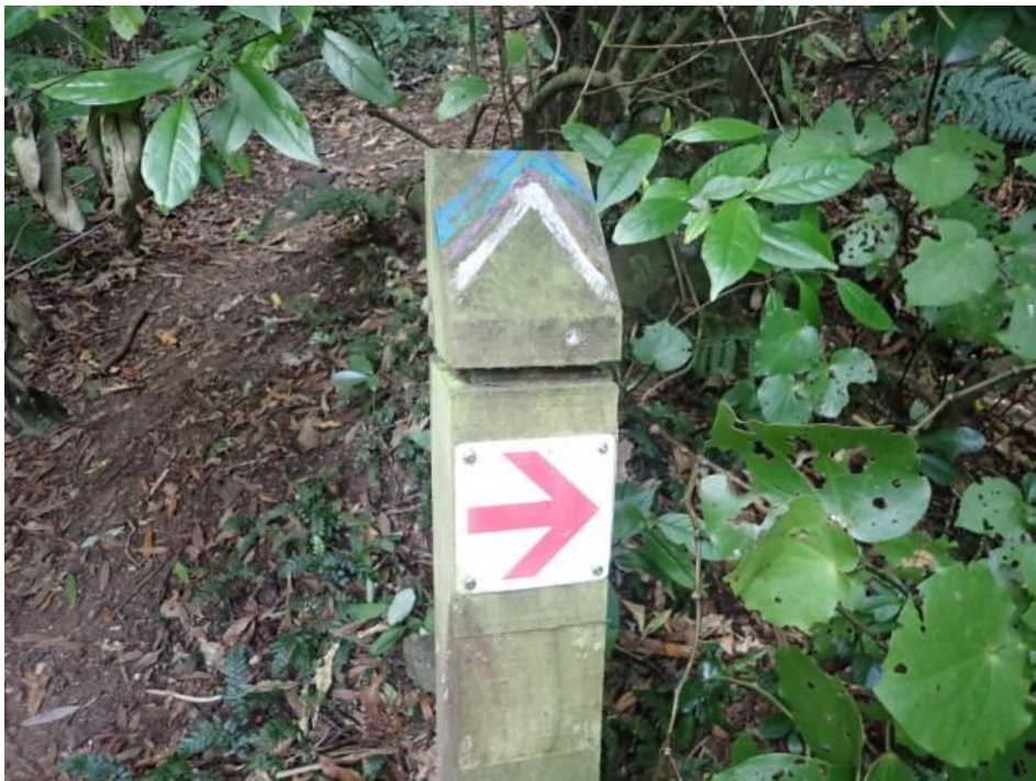
Photo 6: Painted arrow on top of bollard Comment: This points to an old retired track. Also, there is a missing red arrow. Recommendation: Refurbish bollards.
