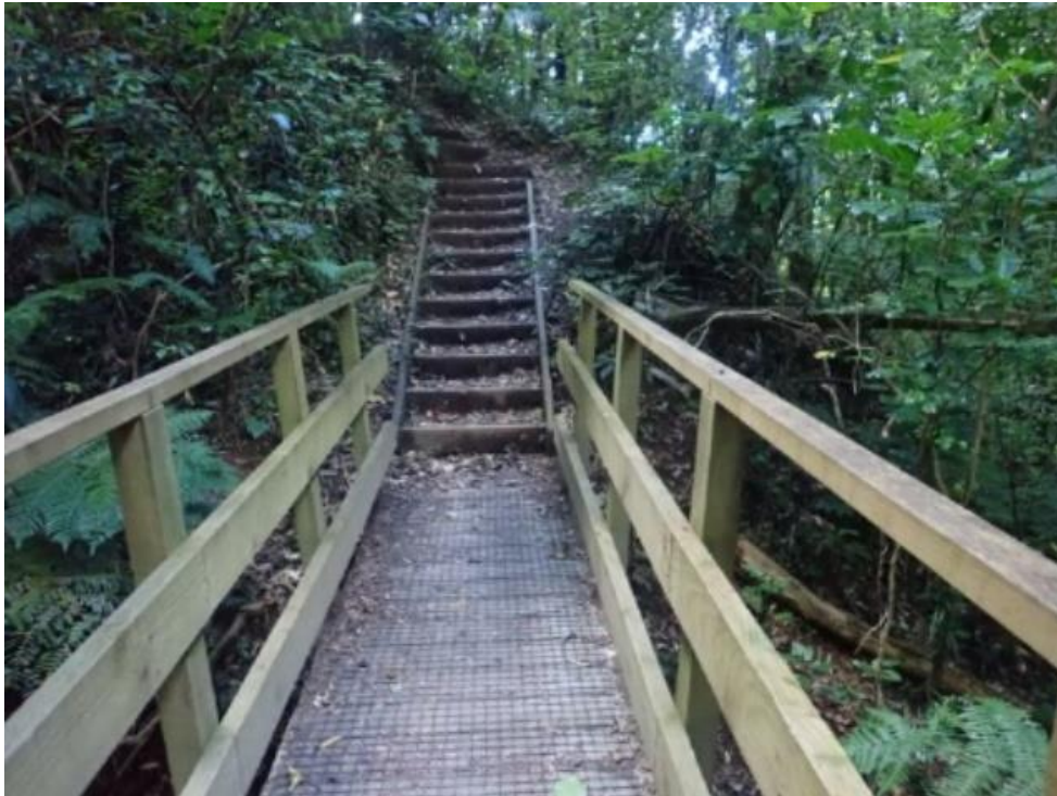
Photo 6: Bridge, 6m by 1.0m with handrails
