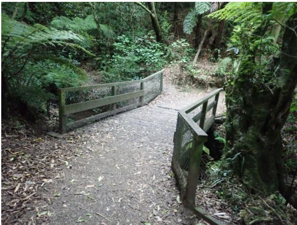
Photo 22: Bridge over side stream
