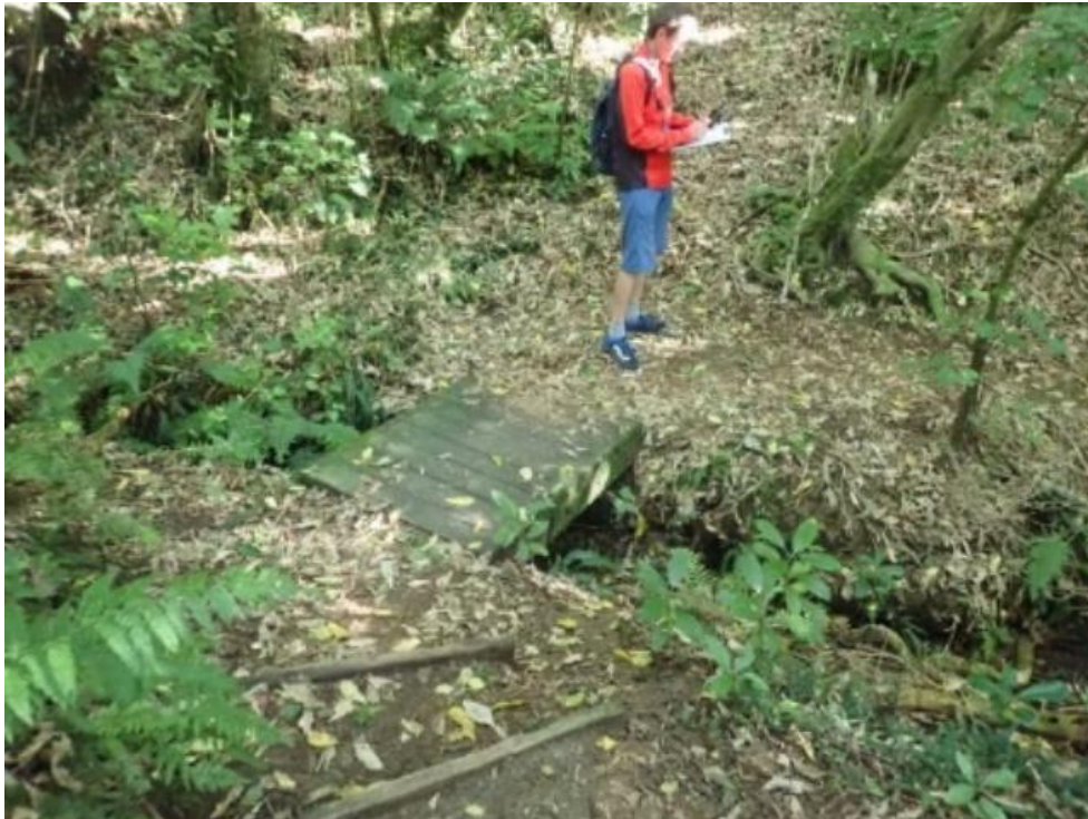
Photo 9: 10 old steps leading to 1.3m by 1m boardwalk
