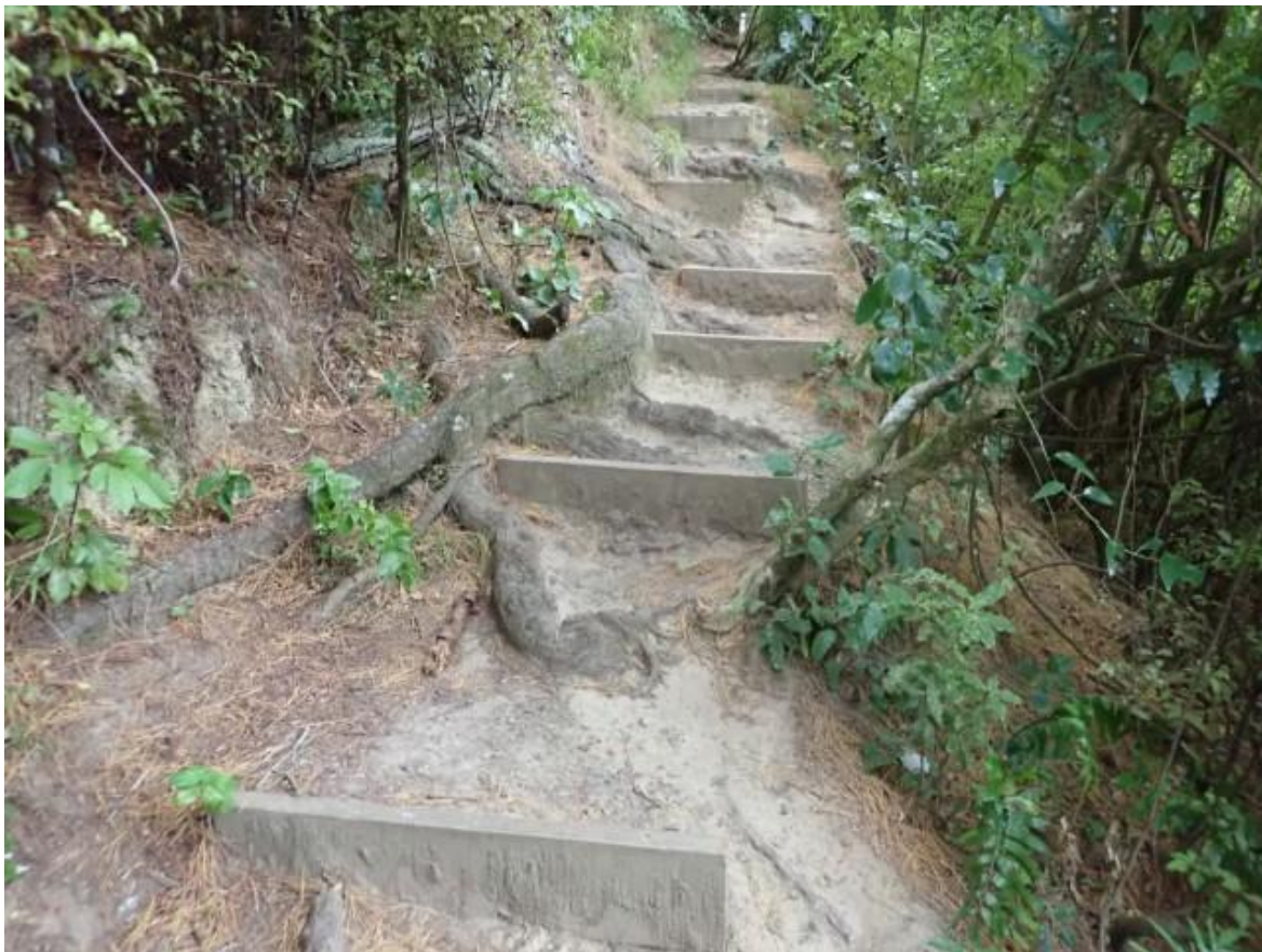
Photo 8: Steps with no backfill material
