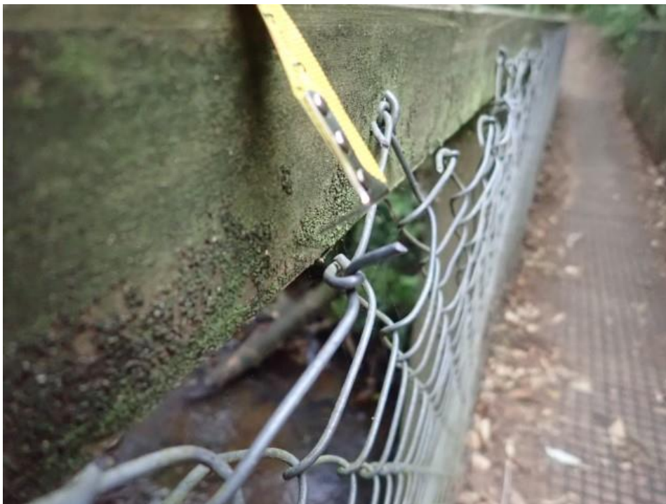
Photo 17: Narrow bridge – 0.78 metres with wire sides
