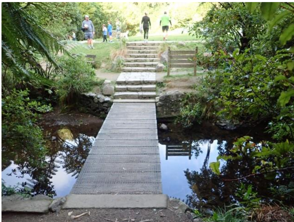
Photo 2: Blue Trail bridge, 4.7m by 1.5m over Kaiwharawhara Stream
