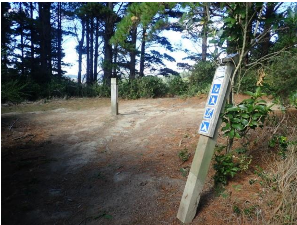
Photo 13: Four tracks meeting at the central bollard and an uprooted sign.
