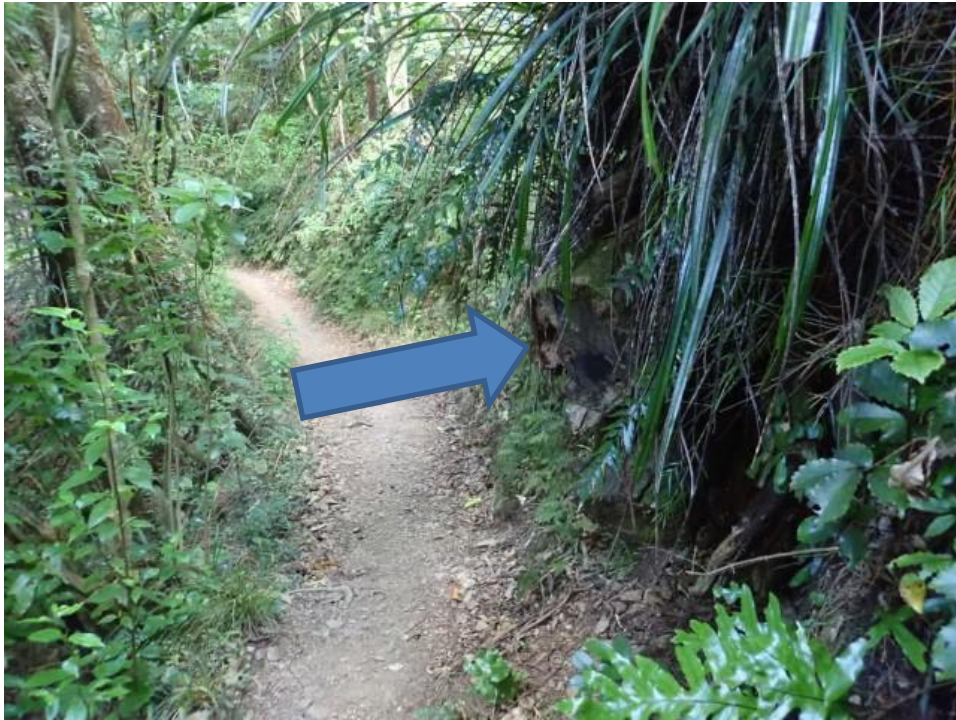
Photo 43: Old tree trunk hidden behind vegetation Comment: This old trunk encroaches on the track corridor. Recommendation: Cut back by 500mm.
