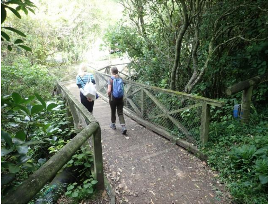
Photo 39: Bridge, 15 by 1.5 metres
