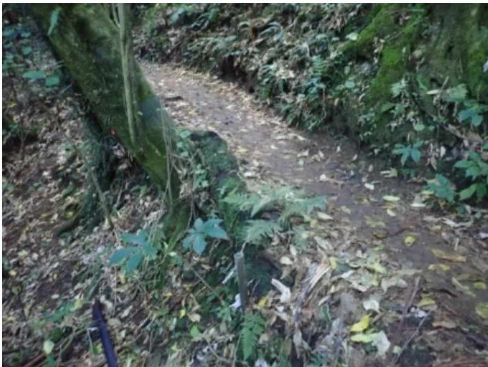
Photo 6: End of 13-metre-long retaining wall
